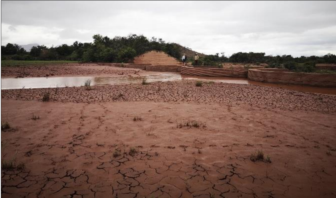
Figure 3-48 Views of the sediment directly upstream of an intervention and the remaining pool of water
