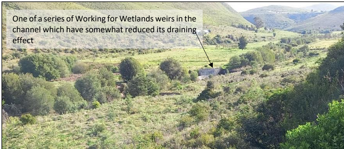
Figure 3-11 The inflow portion of the wetland, highly transformed by agricultural development over most of its surface and with an excavated and incised central channel with invasive alien infestation along its entire length.
