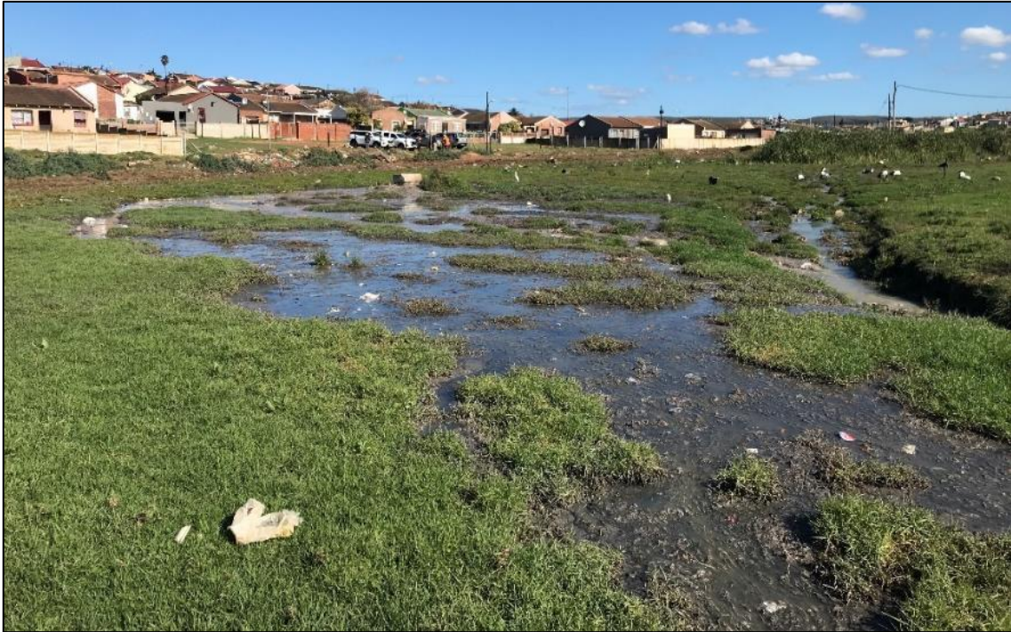
Figure 3-40 A surcharging sewer manhole pictured centrally, and a newly incising channel pictured to the right located in CVB 3. The lateral tongues of the incising channel (heading towards the manhole) and the proximity of the point of incision to this surcharging manhole indicate that this manhole has been a large causal factor in the incision of this channel
