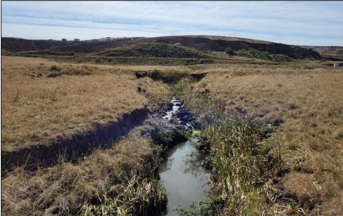
Figure 3-121 Breached dam wall within the valley-bottom wetland. The breach is most likely as a result of the advancing headcut erosional feature.
