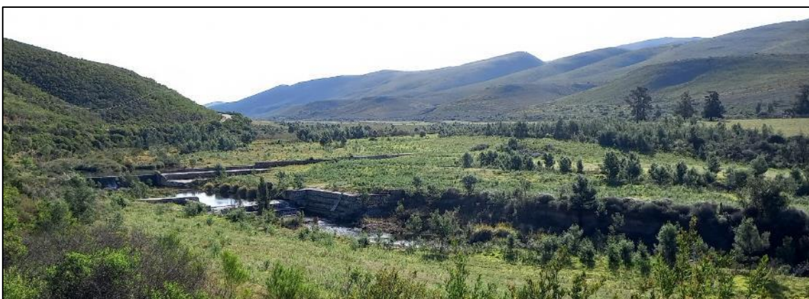
Figure 3-15 Two major rehabilitation weirs lying at the downstream end of the Kompanjiesdrif Basin, and which continue to prevent the headward advance of a major erosion gully threatening the basin's palmiet wetland. Also visible are localized dense infestations of young black wattles
