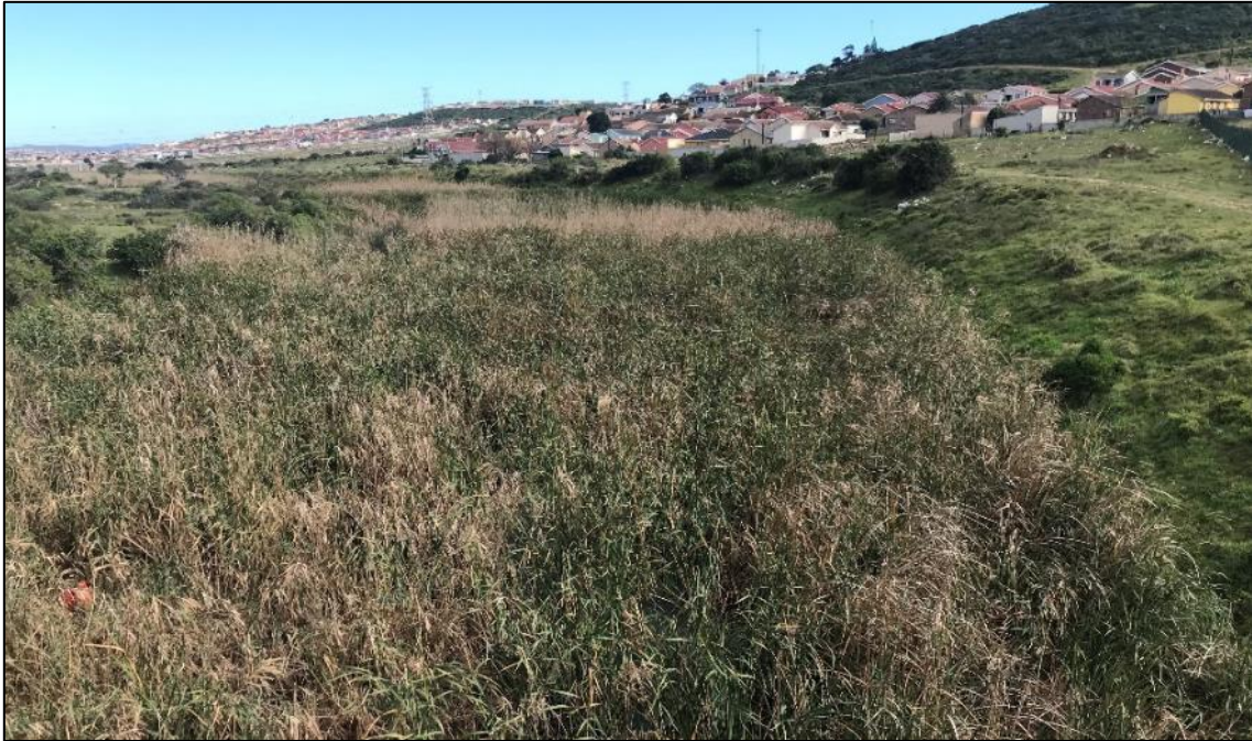
Figure 3-38 Photograph captured from one of the bridges crossing the CVB 1 wetland – with evidence of large scale canalisation of the channel as indicated by the large bank on the right hand-side of the photograph.
