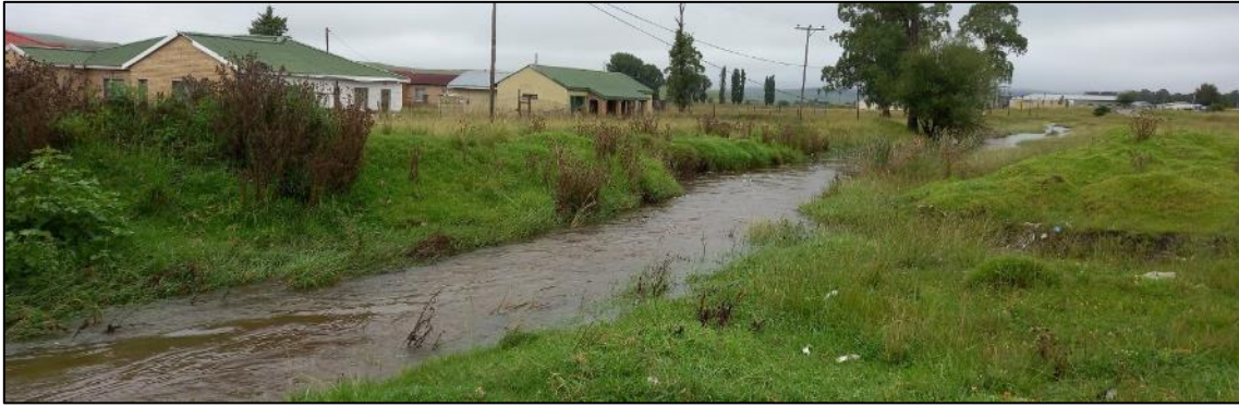
Figure 3-96 Flood-prone houses lying adjacent to the enlarged and straightened channel shown in the previous photo.
