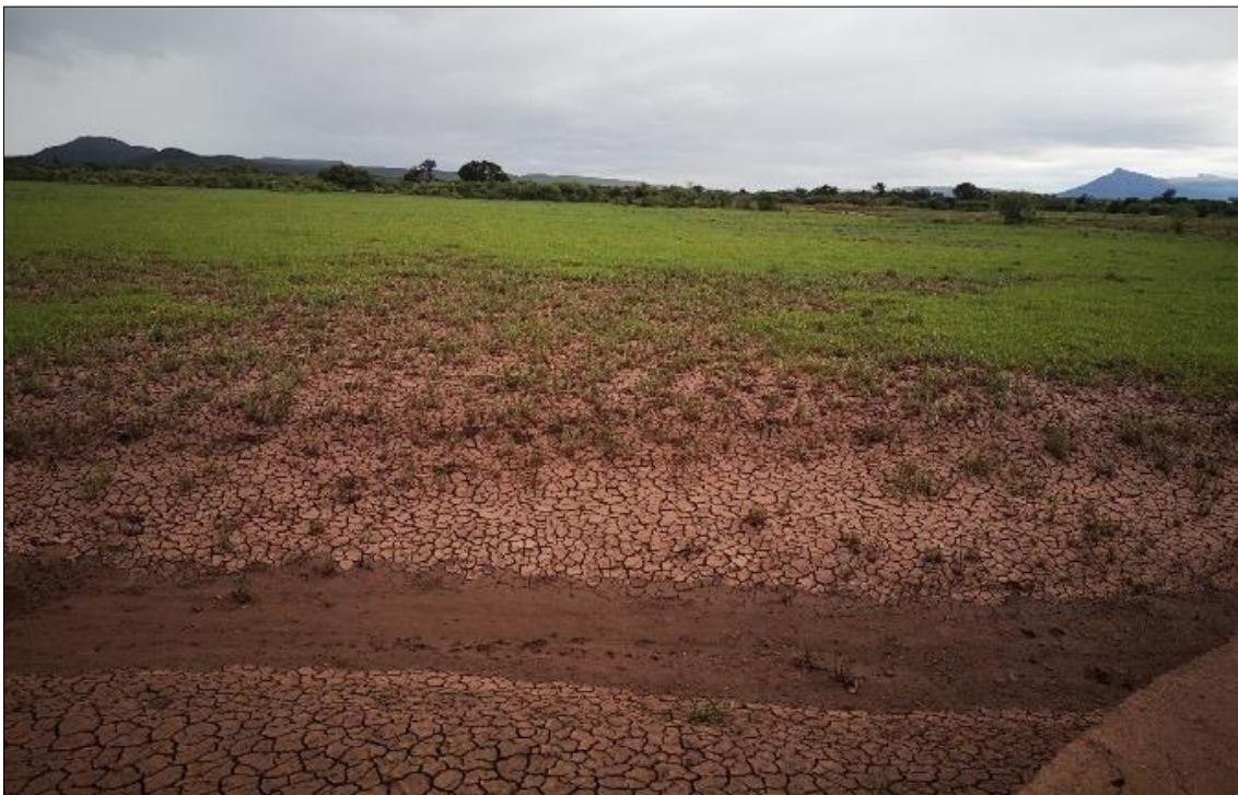
Figure 3-49 View of the accumulated sediment upstream of the weir and heavily grazed grassland
