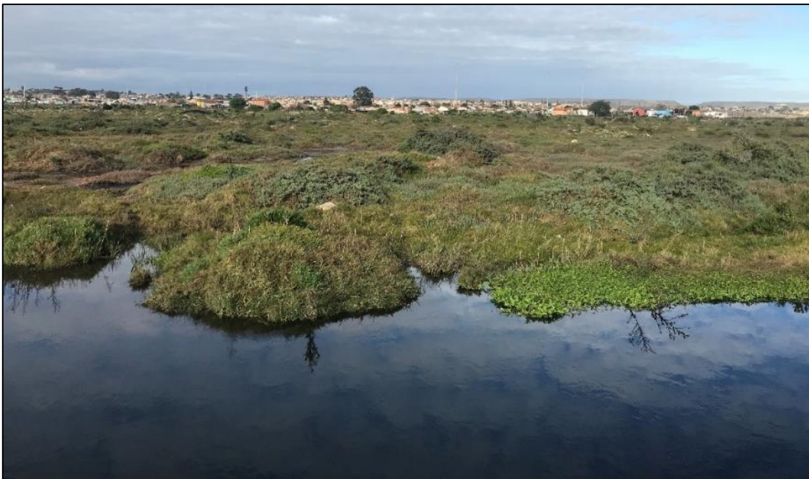
Figure 3-41 Relatively clear and non-odourous water flowing through the toe of the wetland. In addition, this lower section of the system coincided with the most intact vegetation observed across the entire site.
