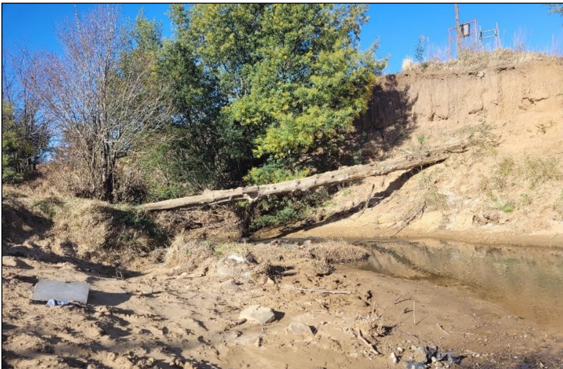
Figure 3-82 Incised river channel within the floodplain, with the discharge point from the waste ponds slightly upstream from this point.
