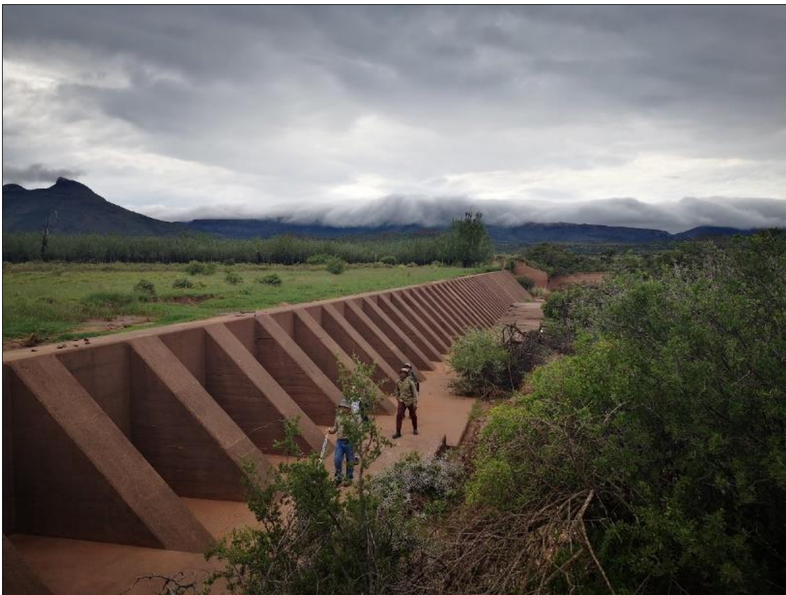
Figure 3-51 View of a buttress weir and the upstream grazing areas
