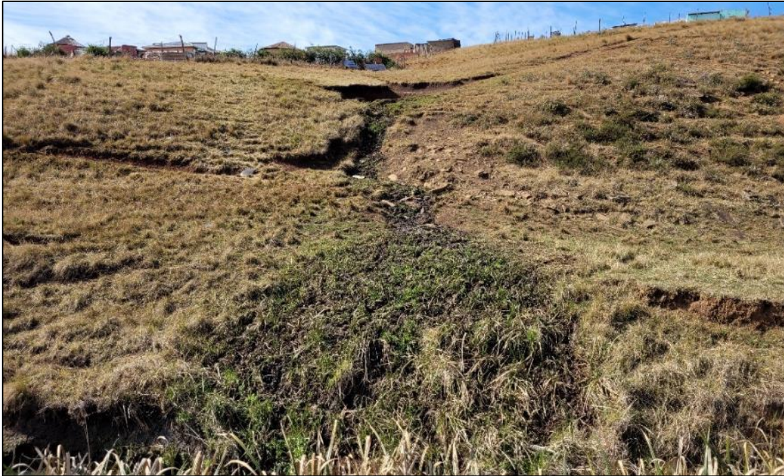
Figure 3-119 Seepage wetland adjacent to the valley-bottom wetland, however, erosional features are present upstream thereof, threatening the integrity of the seepage wetland
